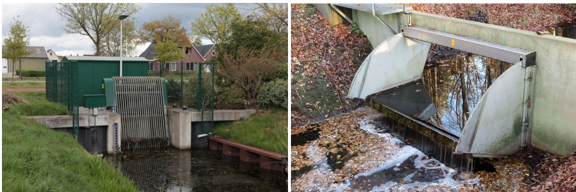
Figure 2.2: A pumping station (gemaal), seen on the left, features a debris screen that can become clogged. On the right, a tilting weir (kantelstuw) is shown. When the water levels rise above the channel, the weir becomes submerged [1].
