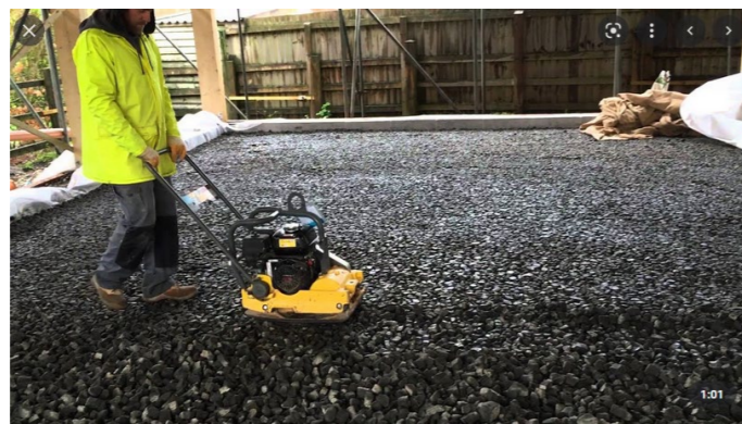
Compacted foam glass
