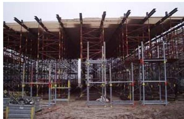
Figure 4.1: Formwork and falsework for deck construction
