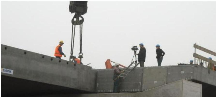
Figure 4.2: Placing prefab beams
