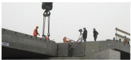
Figure 4.2: Placing prefab beams
