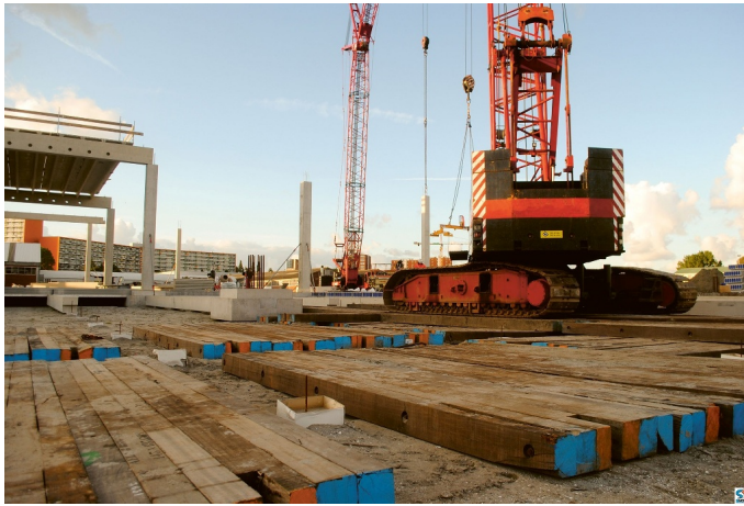
Figure 1.29: Work place created with crane mats.
