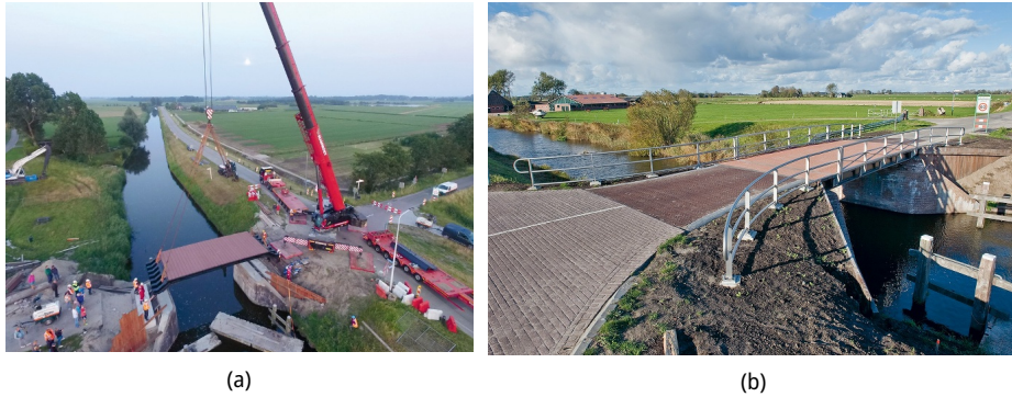
Figure 1.31: Deck profiles of re-used composite at the Dinzer bridge: (a) installation and (b) result (obtained by ten Busschen).
