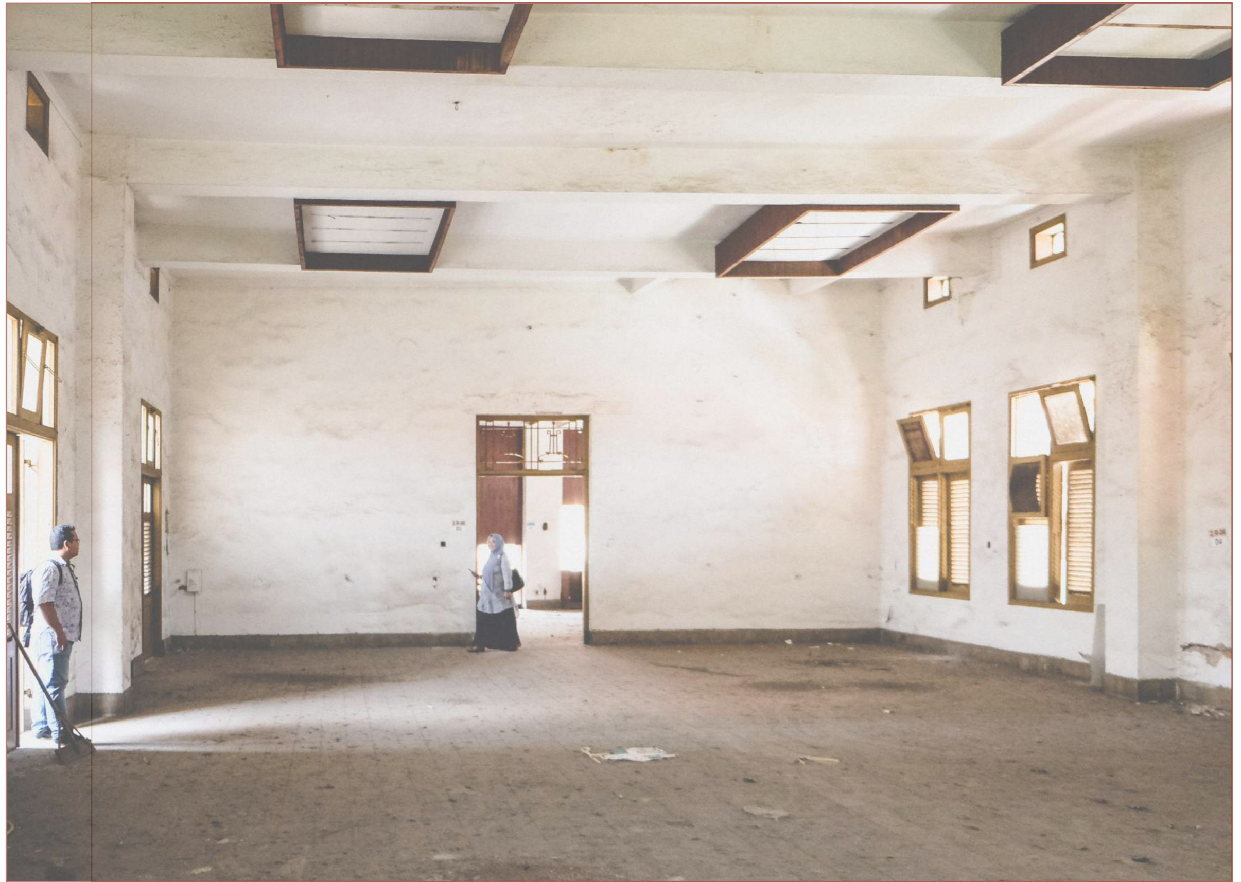
Upper Floor Existing Condition
