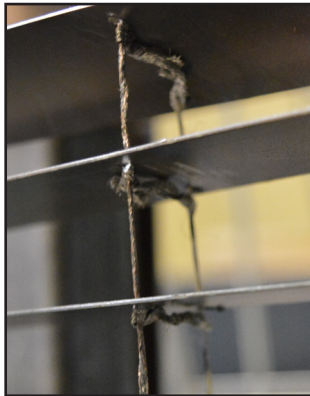
Keeping the lamellae in place by making a metal ladder cord
