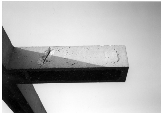
Figure 22: Observed variability of deterioration (Barcelona, Spain, photo by author)
