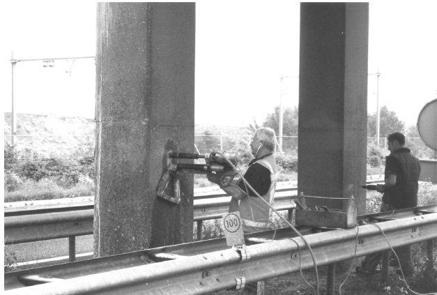
Figure 26: Taking cores from a bridge column (photo by author)
