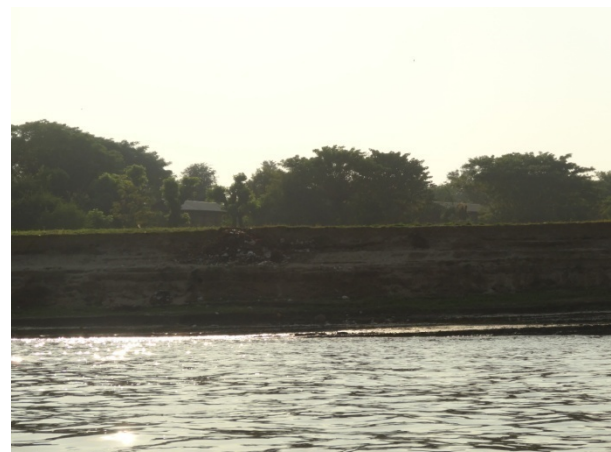
Figure B24 The vegetation on top does not reach the toe of the bank, causing toe erosion to erode the riverbank.
