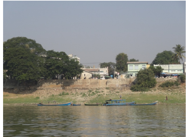
Figure 13 The larger villages need some protections works, like this wall in front of a road. The buildings are in this way protected against the high water levels.
