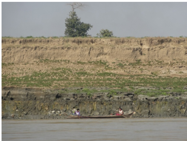
Figure 9 Typical vertical riverbank in the Ayeyarwady. The riverbanks overflow during high water. This bank is classified as a steep riverbank.
