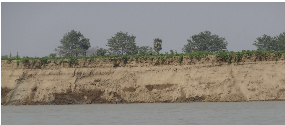
Figure 26 Roots of vegetation are not able to strengthen the soil to prevent mass erosion.
