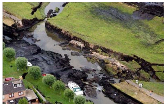
Figure 2.6: Wilnes failure of a peat dike in 2003. https://en.wikipedia.org/wiki/File:Failed_section_of_peat_levee_(Wilnis,_August_2003).jpg
