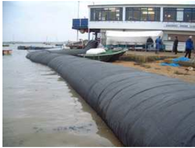
fig. 47 Aqua Dam in action (left) and cross-section with two inner tubes inside outer tube
