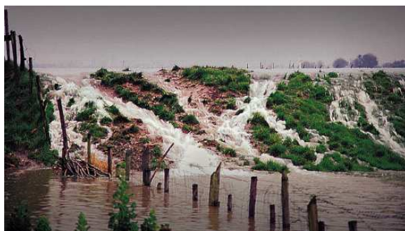
fig. 14 Overflow (left) and macro-instability: slope slide at Streefkerk, 1984 (right)
