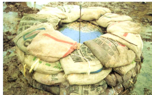
fig. 23 Containment of a sand boil
