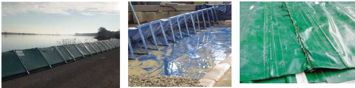
fig. 44 Dutch Convertible Dam (left), Rapidam and the watertight zip of the Rapidam (right)
