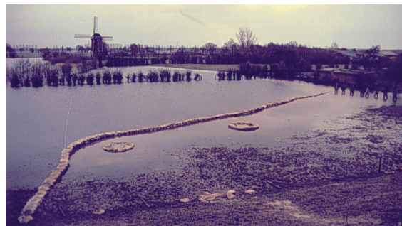
fig. 24 A large scale emergency measure to stop piping
