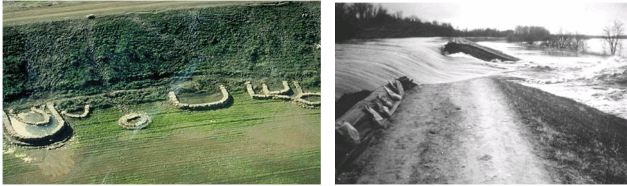
fig. 18 Sand boils and emergency measures in California (left) and a levee breach caused by piping during the 1972 Mississippi flood (right)
