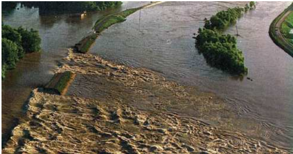
fig. 17 A breached river dike during the Great Flood of 1993
