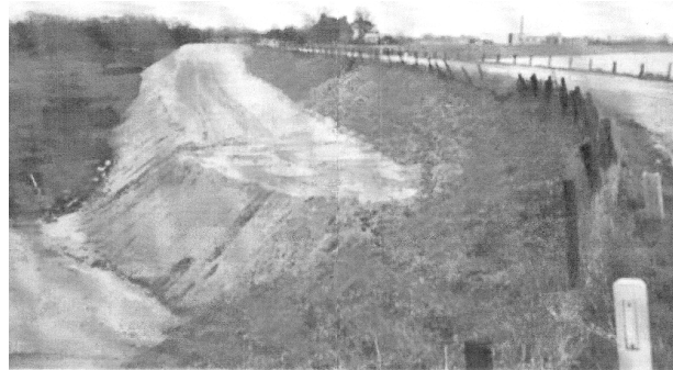
fig. 22 A sand berm along a dike
