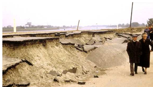
fig. 14 Overflow (left) and macro-instability: slope slide at Streefkerk, 1984 (right)
