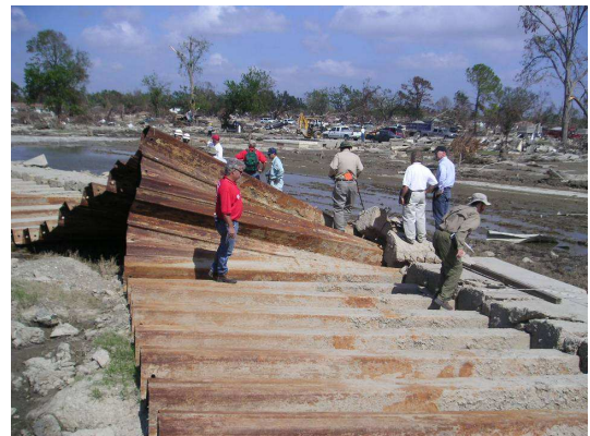
fig. 37 System wall (left) and failure of sheet pile foundation in New Orleans (right)
