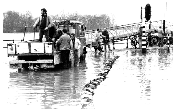
fig. 20 Placing sandbags
