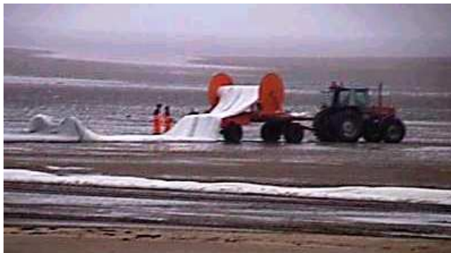
fig. 52 Deployment of the Twin Flex Barrier compared to the Aqua Dam
