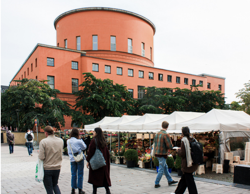
Fig. 17. View on Odengatan. Photograph. Photo: author.
