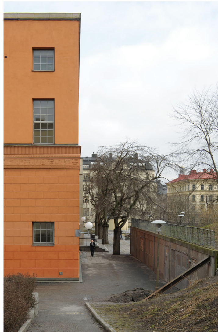
Fig. 24. Exterior view of the South wing corner and passage. Digital photograph. Photo: David Grandorge
