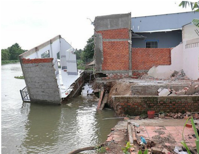
Fig. Two houses damaged due to erosion Photo: Thanh Son
