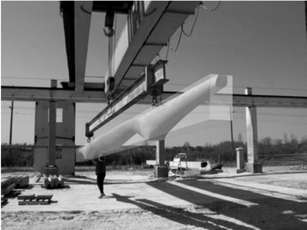
Figure 5.55: Volume of fabric-cast compared to conventional rectangular beam
