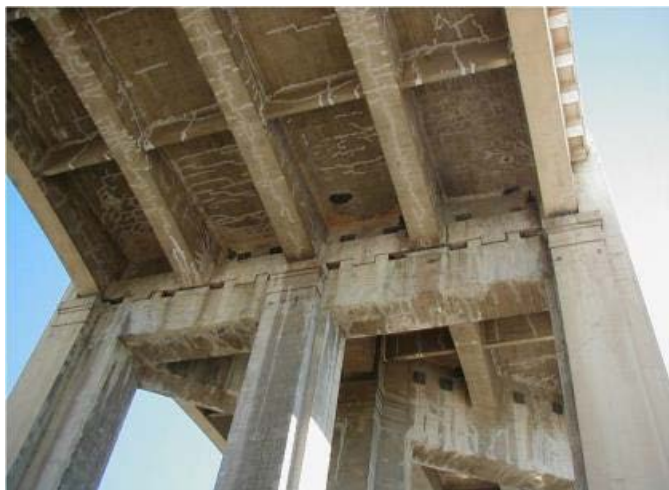
Figure 3.5: Alkali-Silica reaction [CIE5127]
