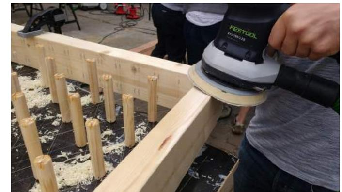
Figure 128: sanding the rough edges of the frame
