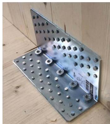
Figure 6.4: TTV Angle brackets [18]
