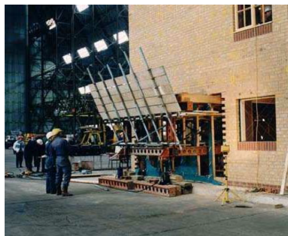
Figure 5.2: Removal outer wall TF2000 [51]
