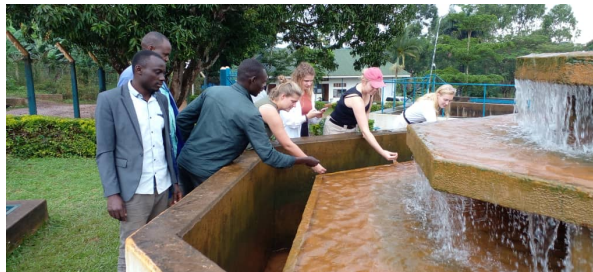
Figure 15.1: Aeration step drinking water treatment plant Hoima
