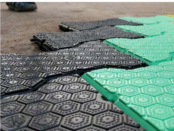
Figure 29 - Street pavers made from recycled plastic
