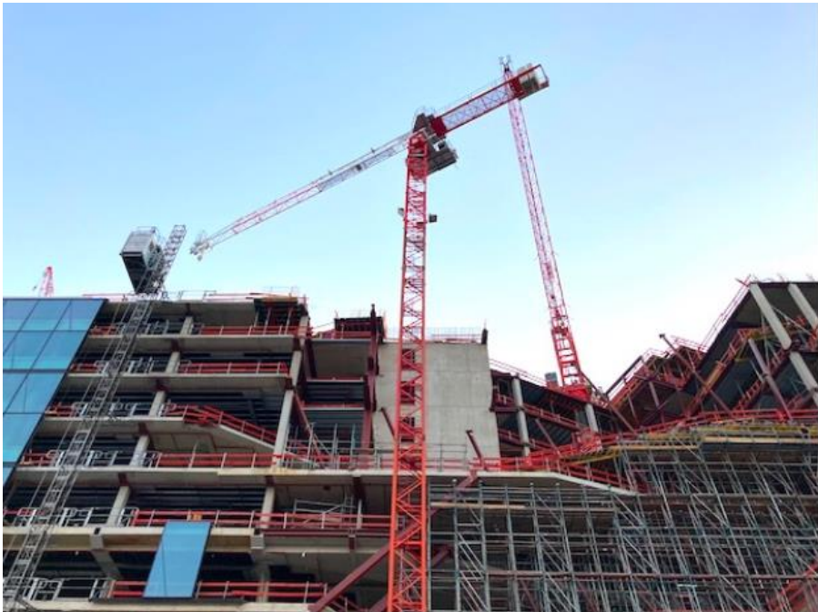
New building under construction Pascoe, R. (2023)
