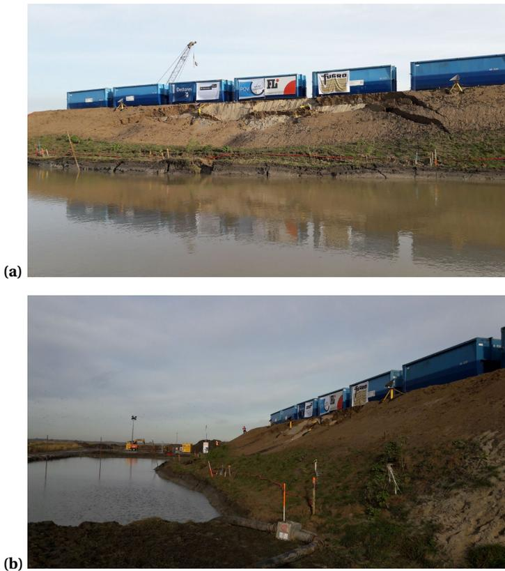
**Figure A.6:** The failure of the green levee.
