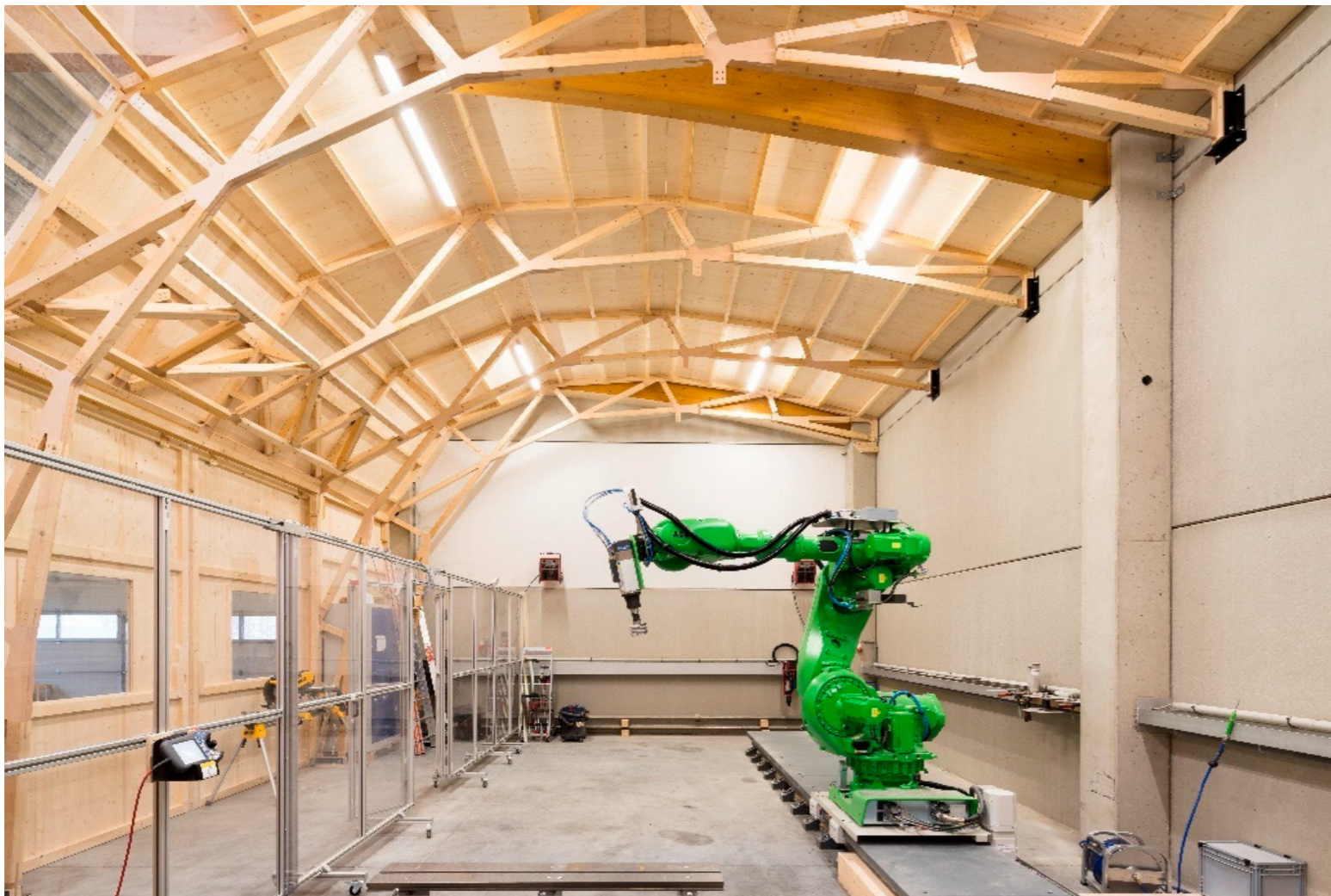
Wooden load bearing structure with wooden nodes (Kromoser et al., 2021)
