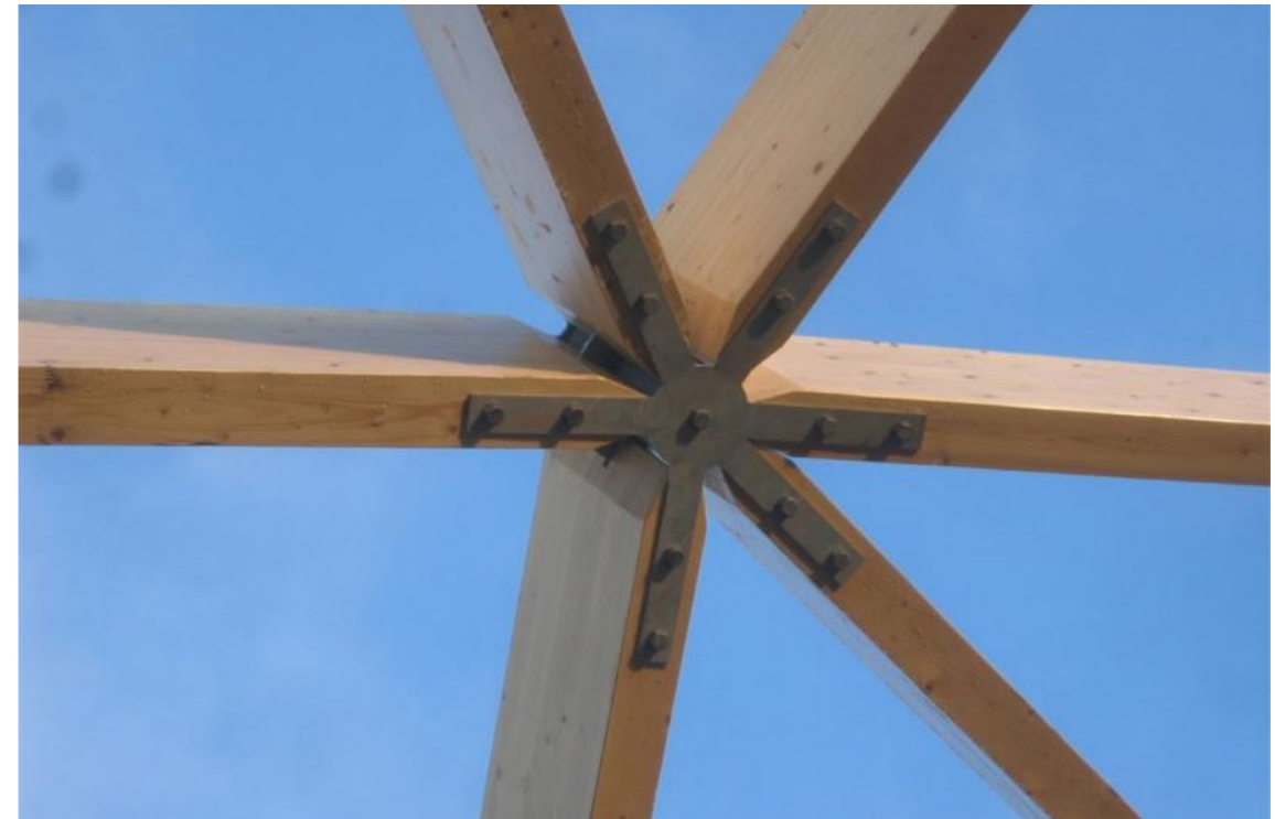
Timber dome canopy, the Jungledome, Remouchamps (Lüning, 2006)
