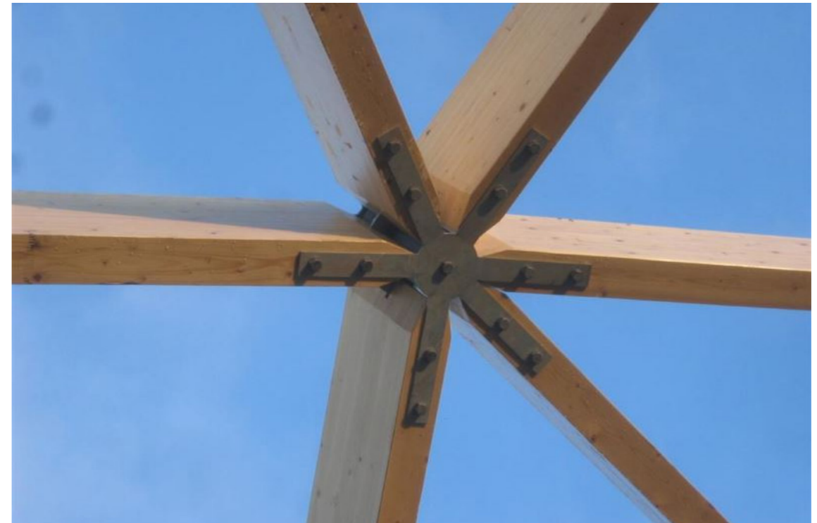
Timber dome canopy, the Jungledome, Remouchamps (Lüning, 2006)
