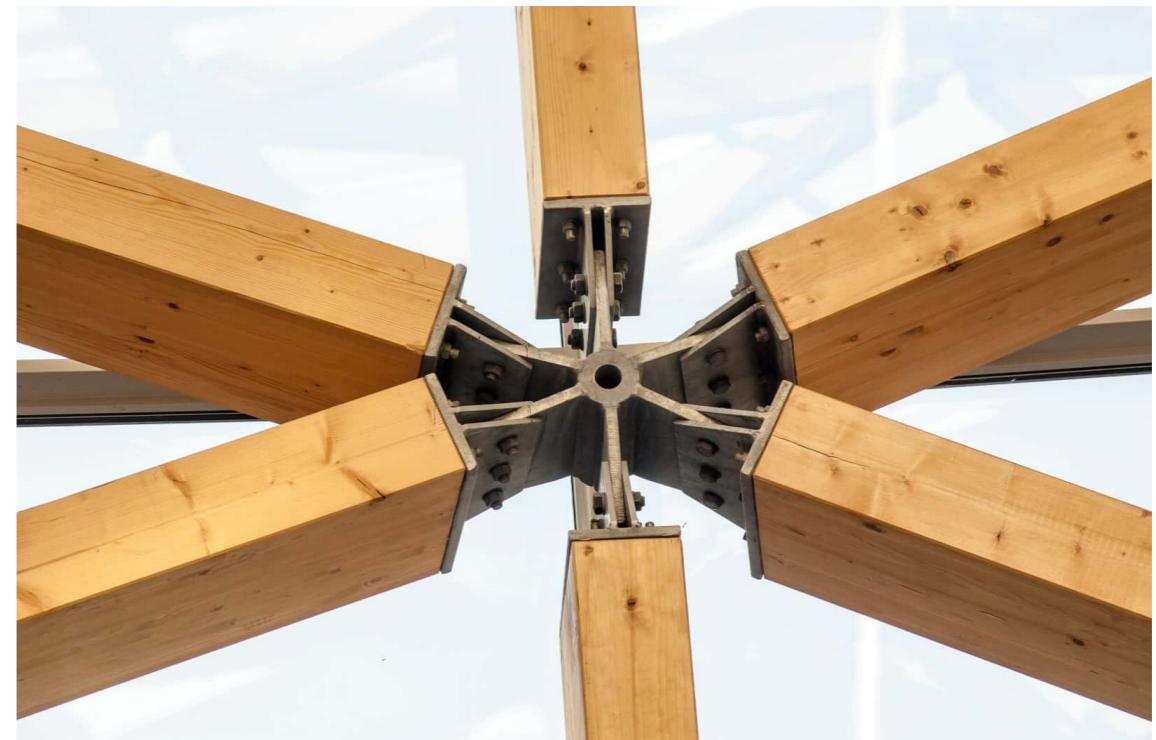
Timber facade structure, The Base, Schiphol-Centrum (De Groot Vroomshoop, 2017)
