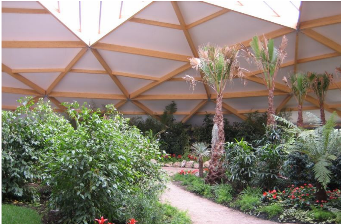
Timber dome canopy, the Jungledome, Remouchamps (Lüning, 2006)
