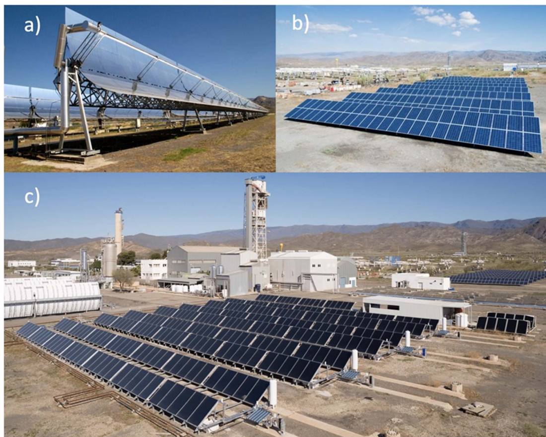
Figure 3. (a) PTC in operation, i.e. a parabolic trough collector used for CSP production. (b) A field of solar PV collectors. (c) A view of a field of stationary flat plate solar collectors that can supply heat at 80 °C.
