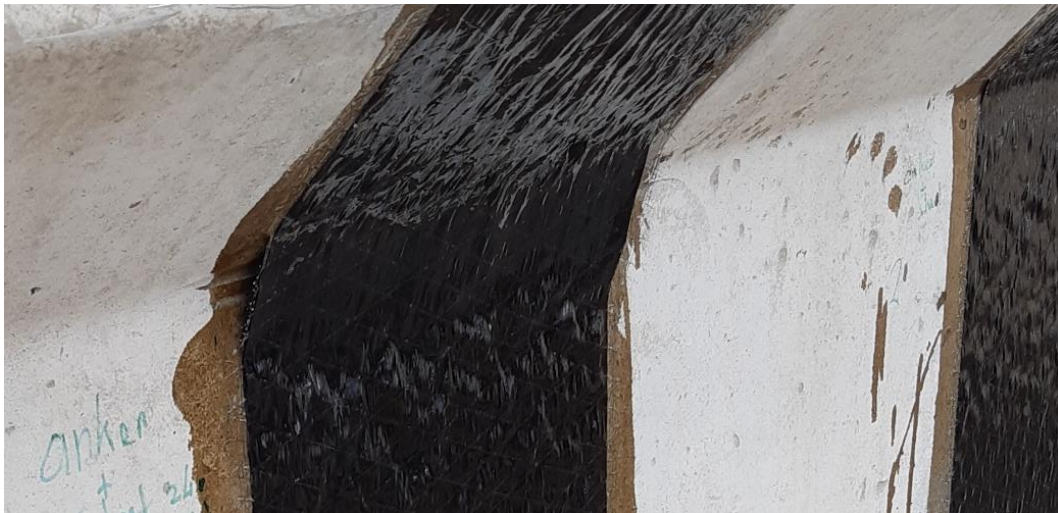
Figure 6.1: CFRP sheet in re-entrant corner (S&P clever reinforcement company)
