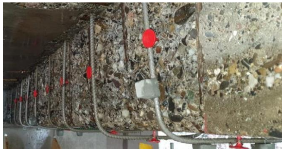
Figure 7.4: Prestressed shear reinforcement Kurtheater baden (Re-fer AG, 2019)
