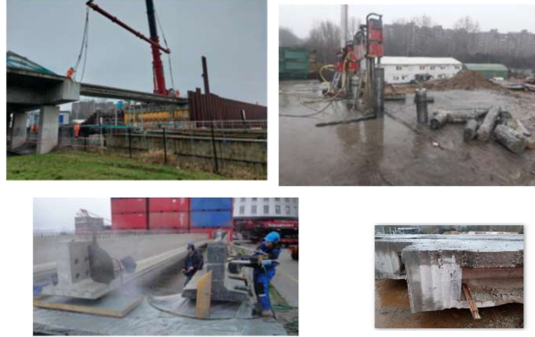
Illustrations of the handling and operations for harvesting prefab concrete beams
