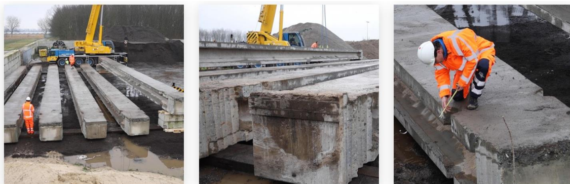
Figure 2.2 Released and reusable prefab concrete beams after 1 st life cycle (Heidinga, 2021)
