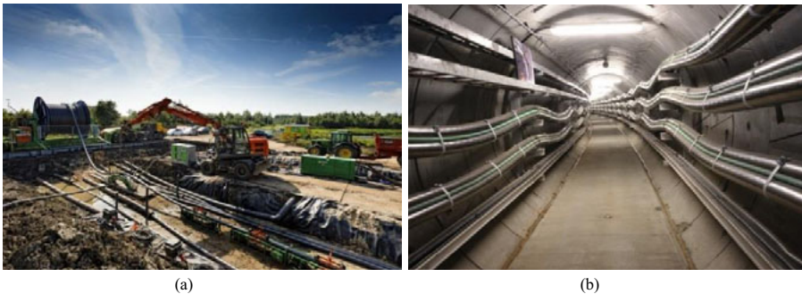
Figure 1.2: Power transmission by underground cables, (a) Randstad 380 kV project in the Netherlands, (b) 132 kV City West Cable Tunnel project in Sydney, Australia.
