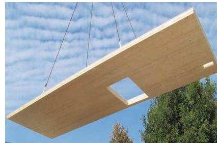
Erection of Cross-Laminated Timber
