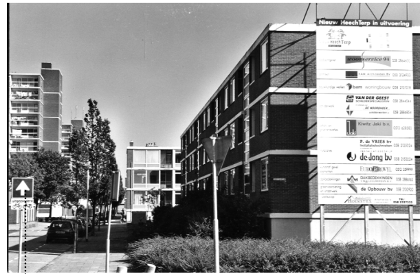
Figure 6. Refurbishment of low rise flats.
