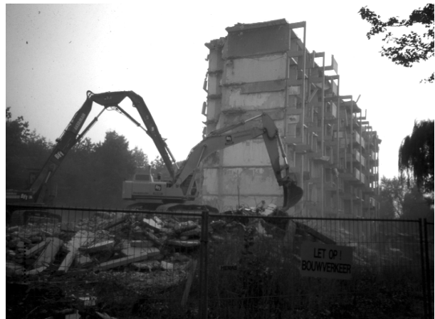
Figure 4. In the Bijlmermeer high-rise district some of the blocks are being demolished and replaced, the remaining are being refurbished.
