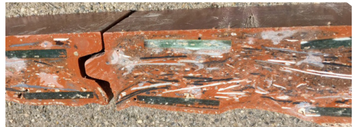
Figure 26: Canal retaining wall (ten Busschen et al., 2016)
