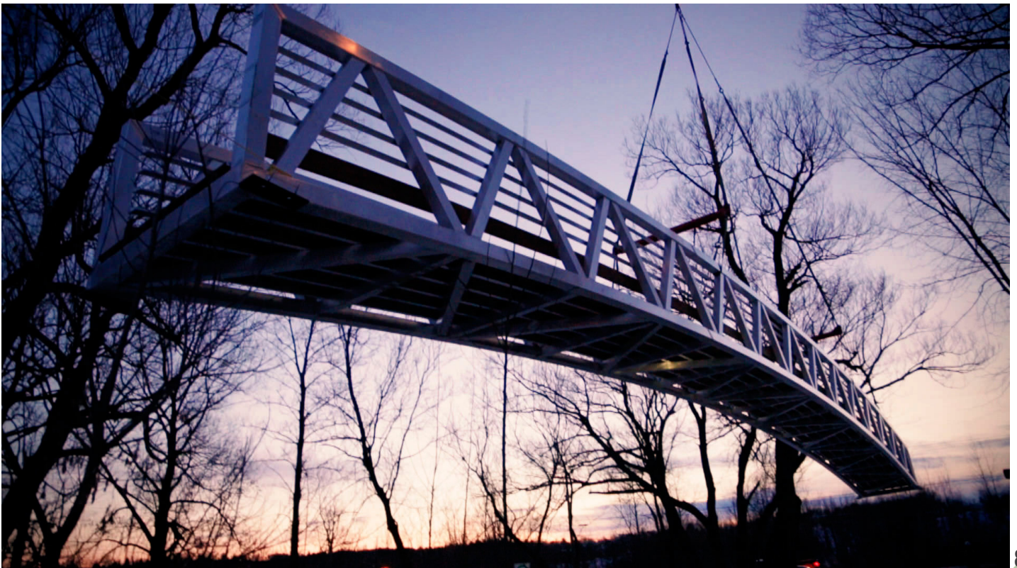
Figure 60: Installation of a prefab bridge.
