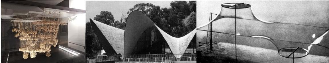
Figure 2-1 Hanging model of Gaudi, Concrete shell of Felix Candela, Soap surface of Frei Otto
