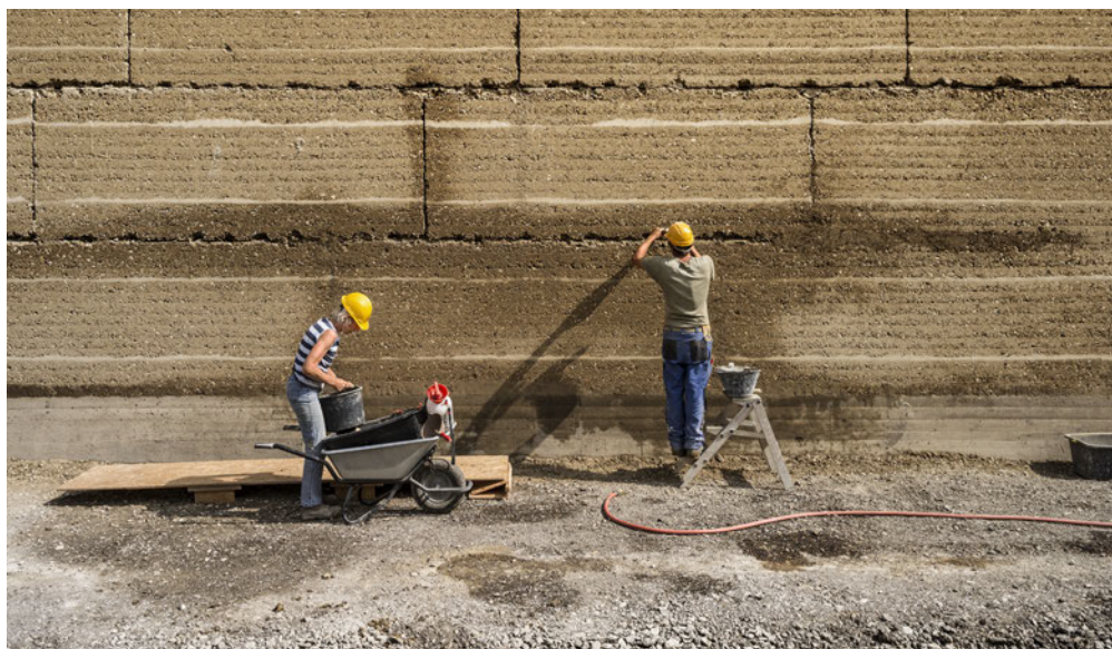
Fig. 25. Retrospective: Martin Rauch, prefabricated rammed earth elements for Ricola Herb Centre [The Architectural Review]
