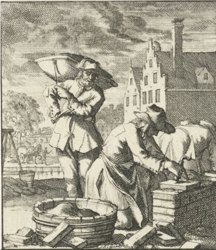
A mason builds a wall of monastery bricks. Etching by Caspar Luyken, after Jan Luyken, from 1694. [Collectie Rijksmuseum]
