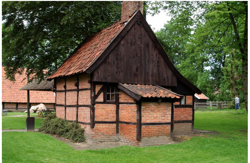
Fig. 4. Timber-framed house filled with bricks instead of rammed earth. (Bakhuuske in Twente) [Hello Oostmarsum]
