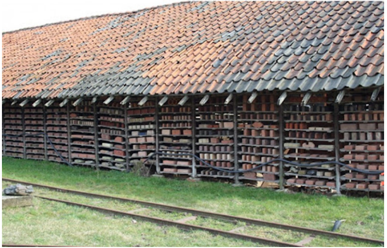
Fig. 3. Architectural Typology of Brick Drying huts (so-called Haaghutten) [Nederlandse Museummaterieel Database]
