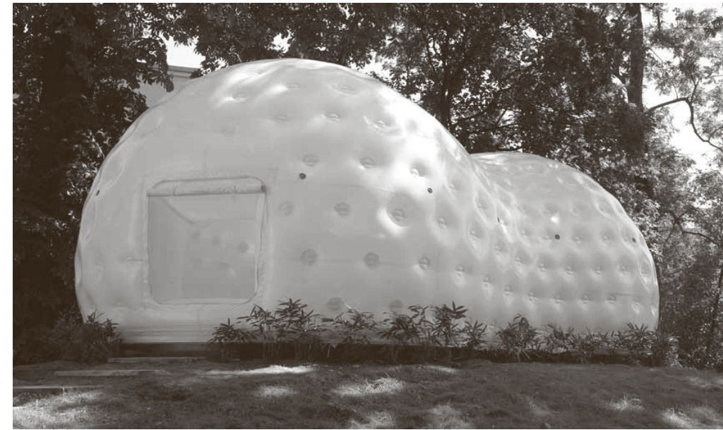
4 Inflatable Tenara Teahouse, Museum für Angewandte Kunst, Frankfurt [Kengo Kuma & Associates]
