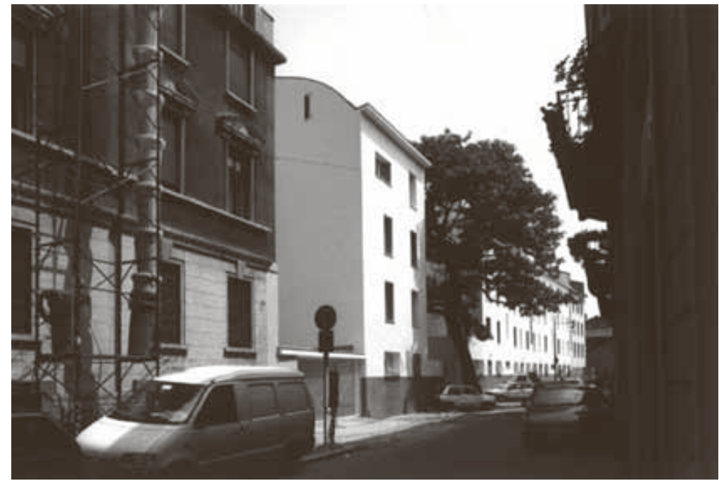
5 Studio Albori, Residential building in Via Altaguardia, Milan, 1993-99, [Gianni Berengo Gardin]
