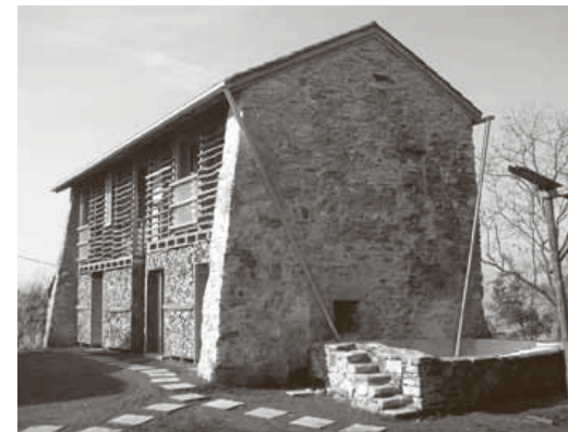
6 Studio Albori, Farm building renovation, Ispra, 2010. [Studio Albori]
