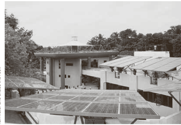
3 WGM TV & Media Center, Battaramulla, Colombo, Sri Lanka, Harald N. Røstvik and Kahawita De Silva Ltd.; in addition to generating electricity, the solar PV system also helps collect rainwater and shade the roof. [Harald N. Røstvik]
