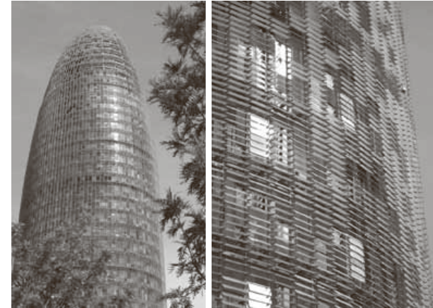
4 Jean Nouvel's Torre Agbar in Barcelona, Spain; the tower employs an intricate system of operable translucent louvers that regulate the natural ventilation of the façade. [Harald N. Røstvik]
