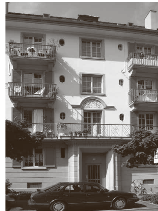
3 A typical street facade with one entrance door after the renovation in 2006. [Marie Antonette Glaser] 4 The original doors from the kitchen to the balcony with a view to the street. [Annelies Adami]
