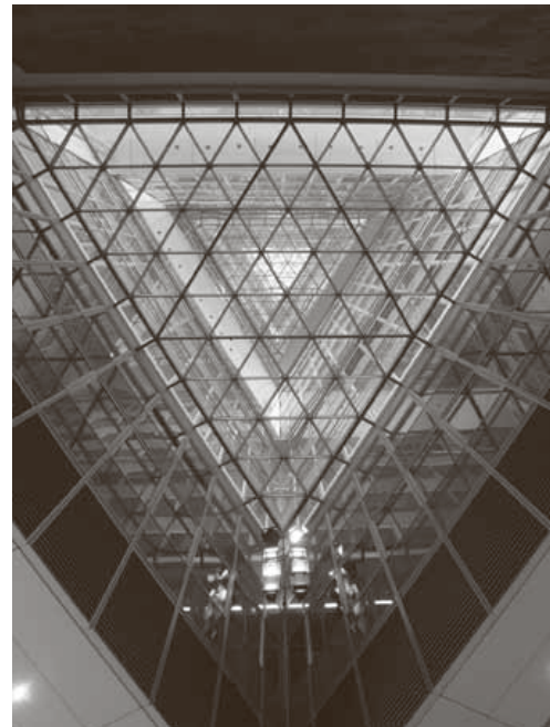
7 California Academy of Science, San Francisco (Renzo Piano Building Workshop). [RFBW, Nic Lehoucq] 8 Commerzbank Headquarters, Frankfurt (Foster & Associates). [Luca Fincicchio & Anne Grete Hestnes]
