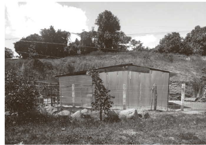
5 A so-called microwave, a low-income housing structure with the roof and walls constructed from corrugated metal sheets in El Salvador, 2004. (Gabriel Arboleda)
