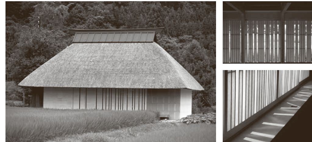
1 Takayanagi Community Center, [Mitsumasa Fujitaka, HELICO Co., Ltd.] 2/3 Interior View/Light Effect of the Washi Screen, [Mitsumasa Fujitaka, HELICO Co., Ltd.]
