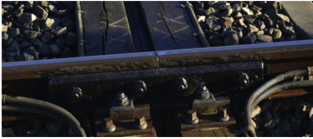
Fig. 21. Typical IRJ in the Dutch railway network.
