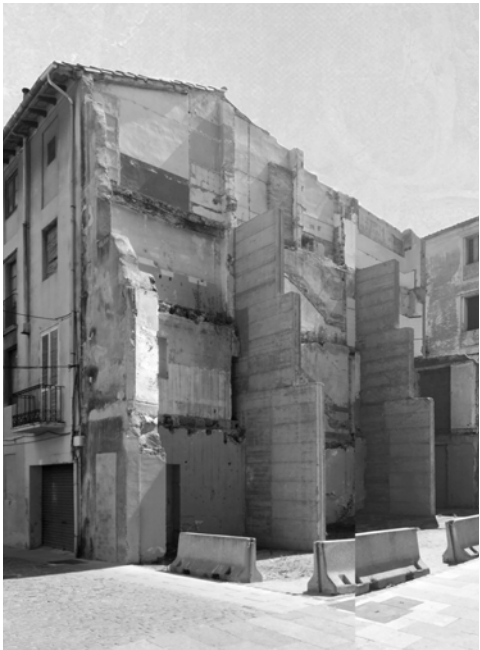
Figure 8. Exposed buttresses and partial wall.
