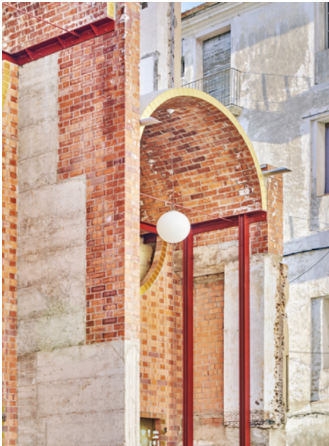
Figure 9. Material layering showing the history of interventions.
