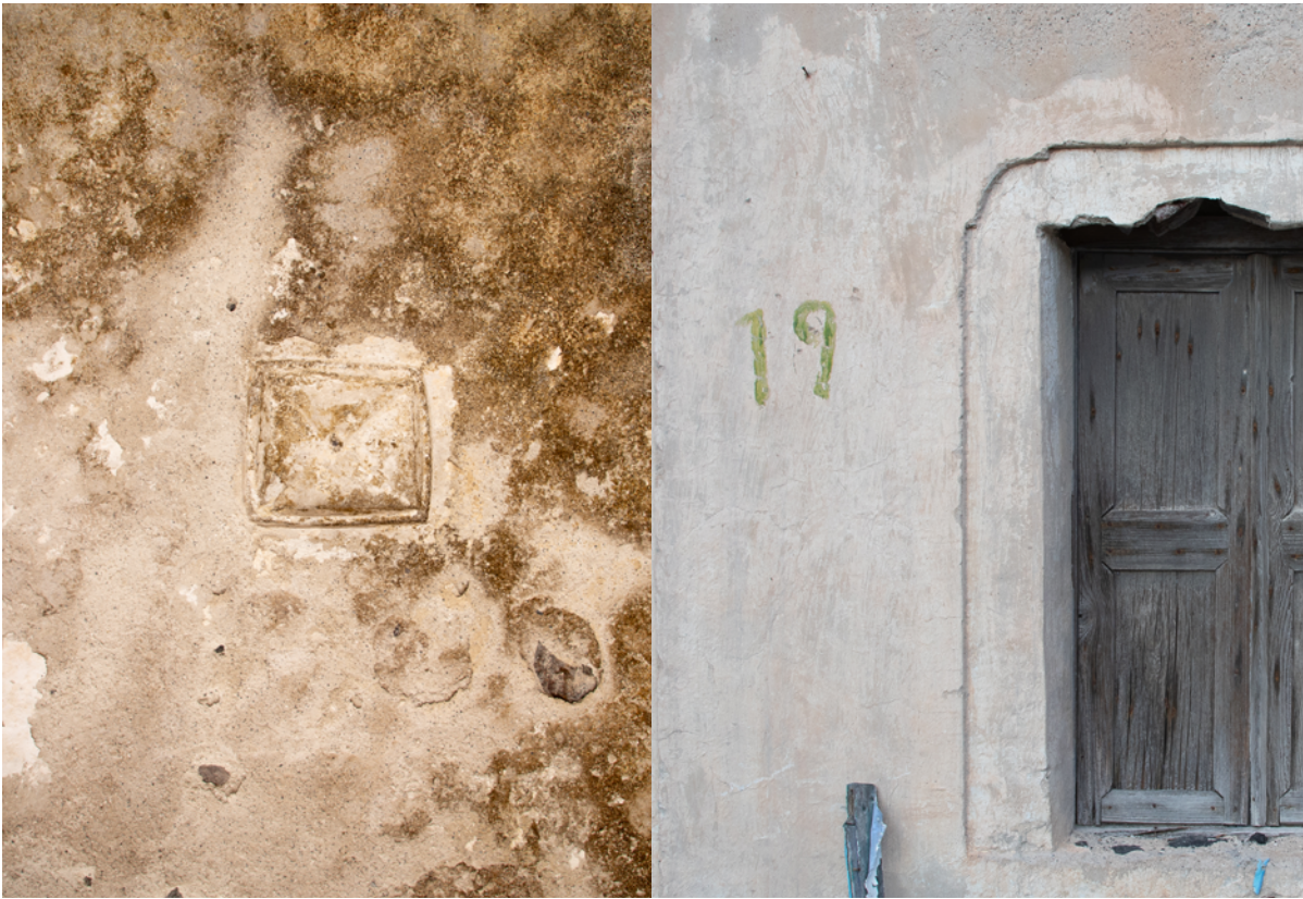
Figure 130. Light fixture and window details, showing the versatile plasticity of Theran earth when mixed with different quantities of lime.
