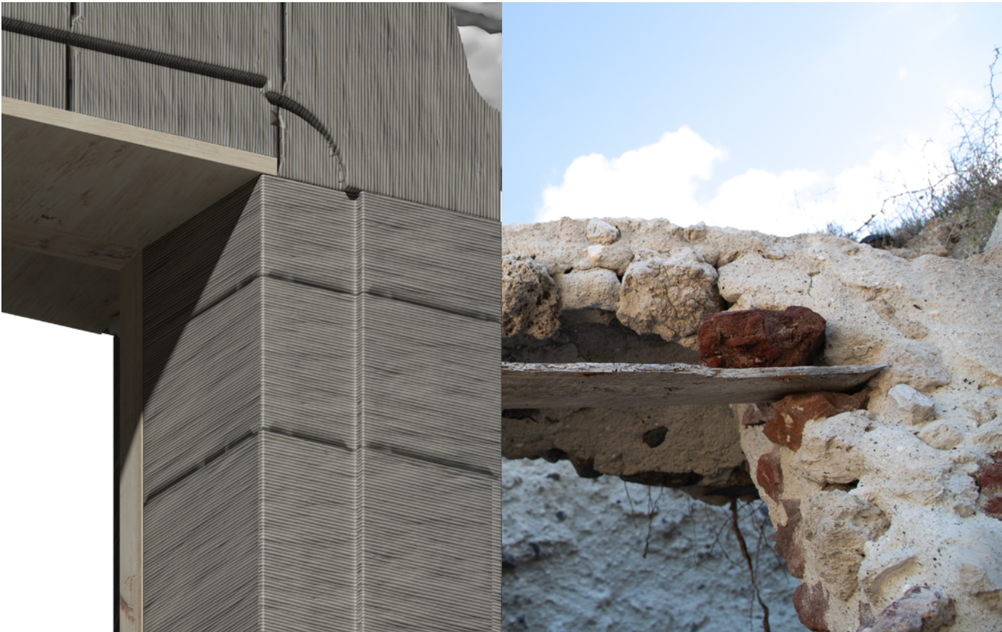
Figure 151. Detail of integrated lintel next to an actual integrated lintel in Agrilia.
