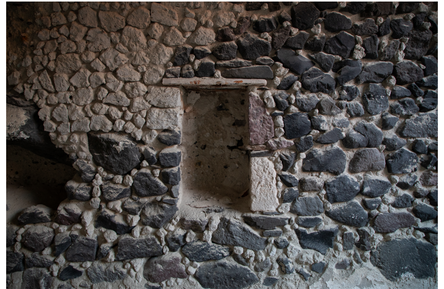
Figure 123. Interior wall with shelf. Stones around the shelf are arranged almost randomly creating an intricate abstract mosaic.
