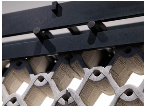
Figure 78. Mounting detail with integrated supports.
