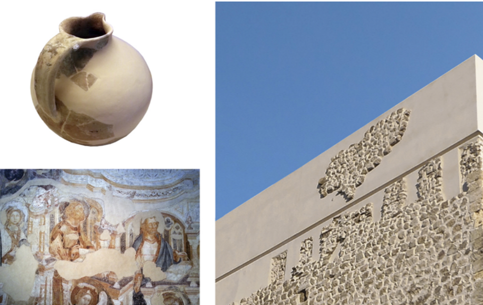
Figure 21. Translation of repair techniques used in art restoration to monument restoration.
