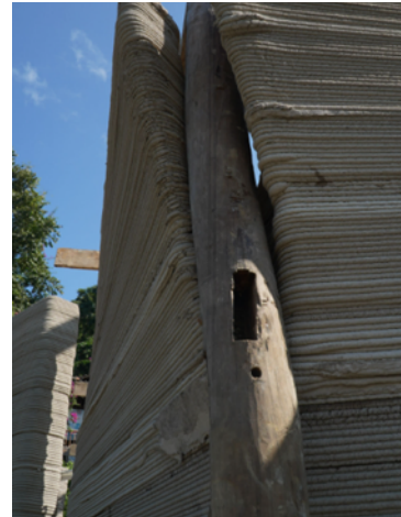
Figure 85. Detail of 3DCP structure wrapped around one of the columns.
