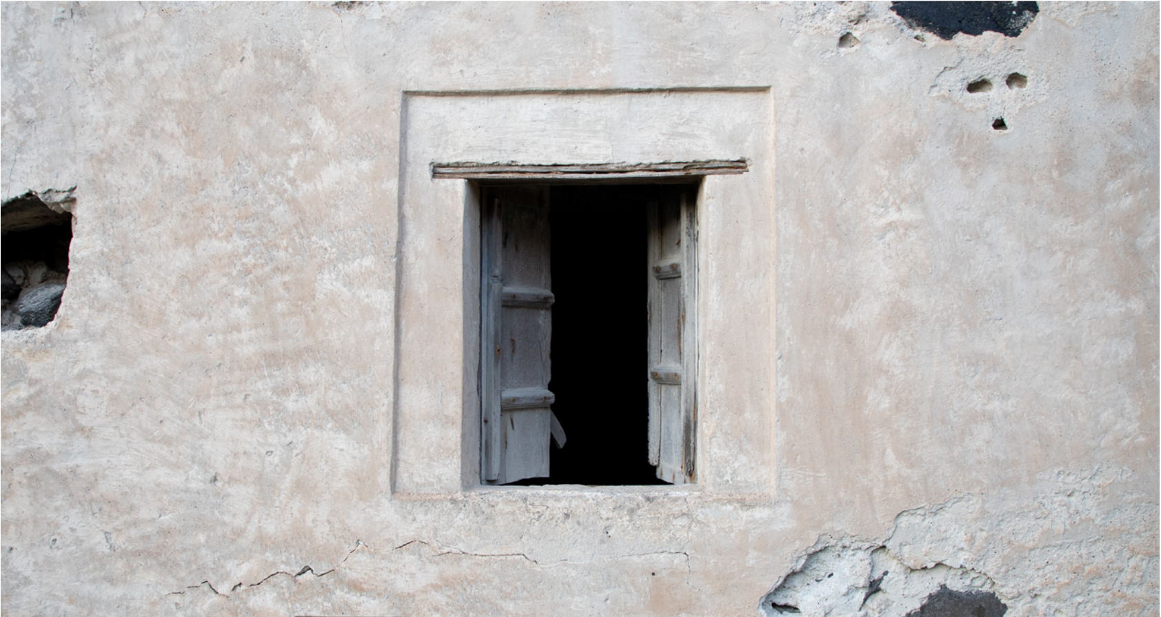
Figure 134. Intact window in Agrilia, showing the complete decorative frame around the window, as well as the wooden lintel as an integrated support element.
