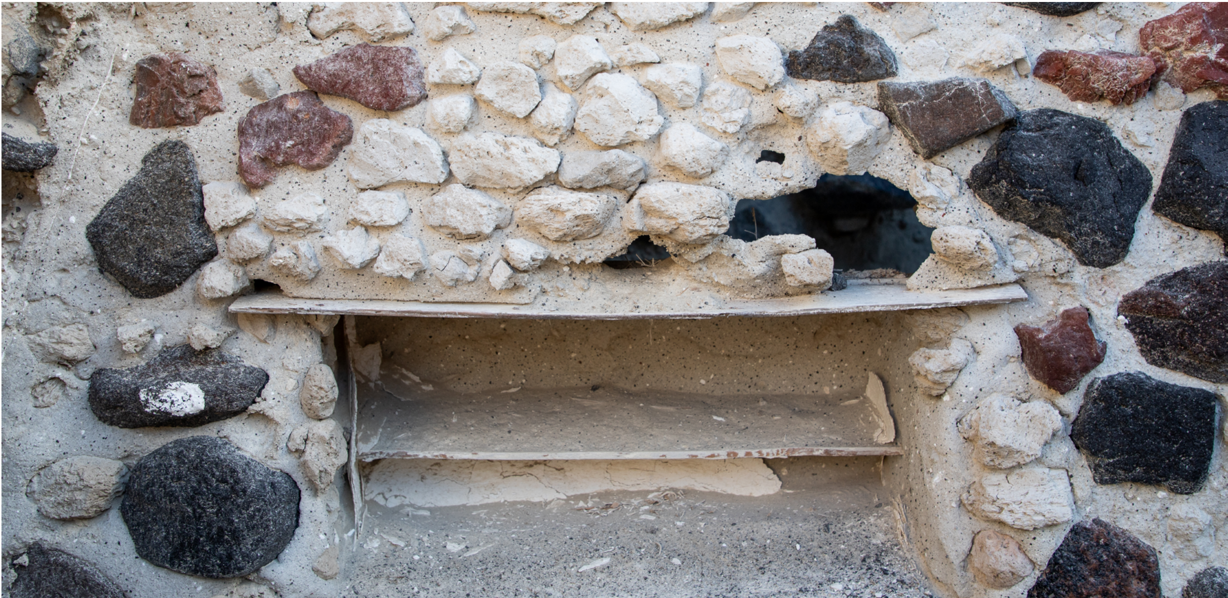
Figure 159. Pumice stone lintel in an interior partitioning wall. In this case, an auxiliary wooden lintel distributes the weight of the stones across the side walls. However, we can observe in its decay that the pumice stone, with the help of mortar, is hanging above the shelf and supporting all of its own weight without weighing on the wood.
