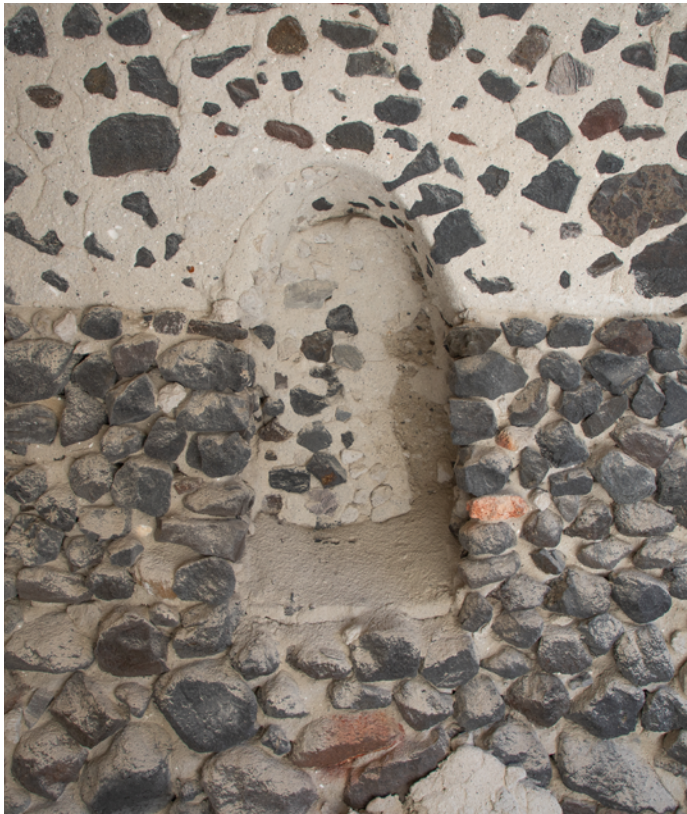
Figure 125. Inside a Theran house, the lack of plaster and limewash reveal the secret to unreinforced domes: Theran mortar.
