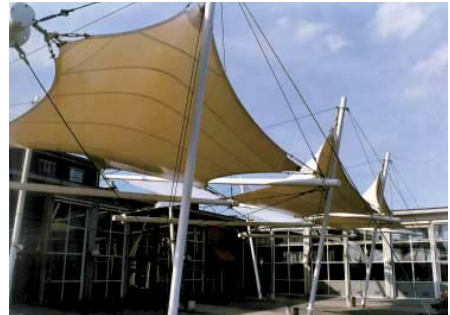
FIG. 33 Realised tensegrity structure with streeked membranes as really built
