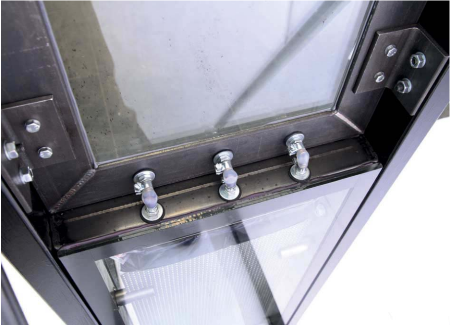
FIG. 79 Airtight connection between cavity and flexible bag
