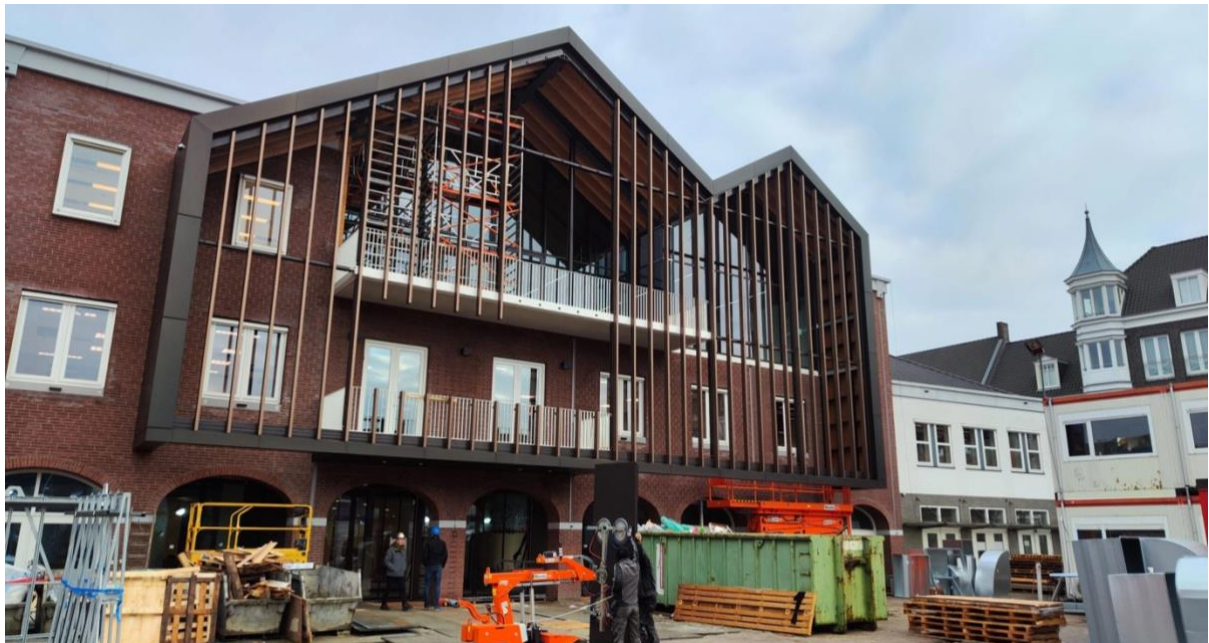
Figure 15: Bruis during execution (Group A, 2025).
