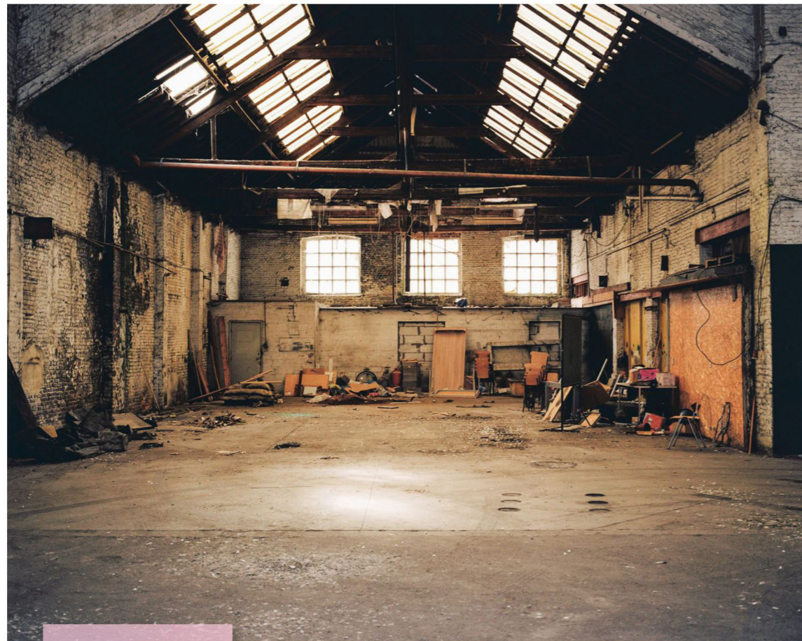
existing conditions inside the hall
