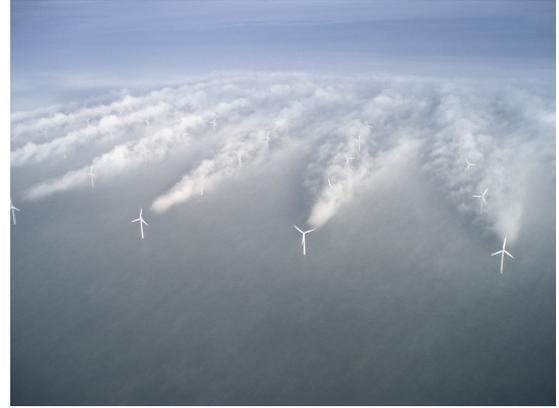
**Figure 8.2:** Photograph of the Horns Rev wind farm showing wake effects visualised by local condensation. Photo by Steiness [52].
