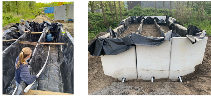
(a) Installation of underdrains. (b) Gravel, coarse sand, and fine sand filled.
