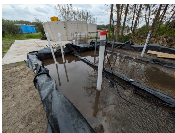
(a) Swale #3, filling attempt.
