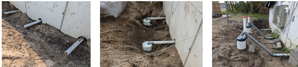
(a) Outlets of underdrains.
