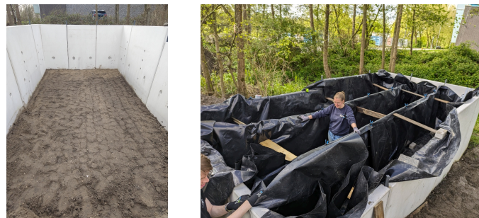
(a) Base layer with 2% slope. (b) Securing plastic lining over wood planks.
