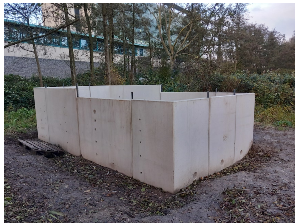
Figure 2.1: MeSUDa facility at start of current project
