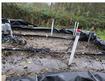
(b) Swale #1, tracer testing.
