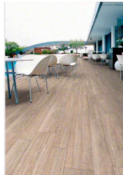
Exterior Floor: Porcelain Wood Tile
