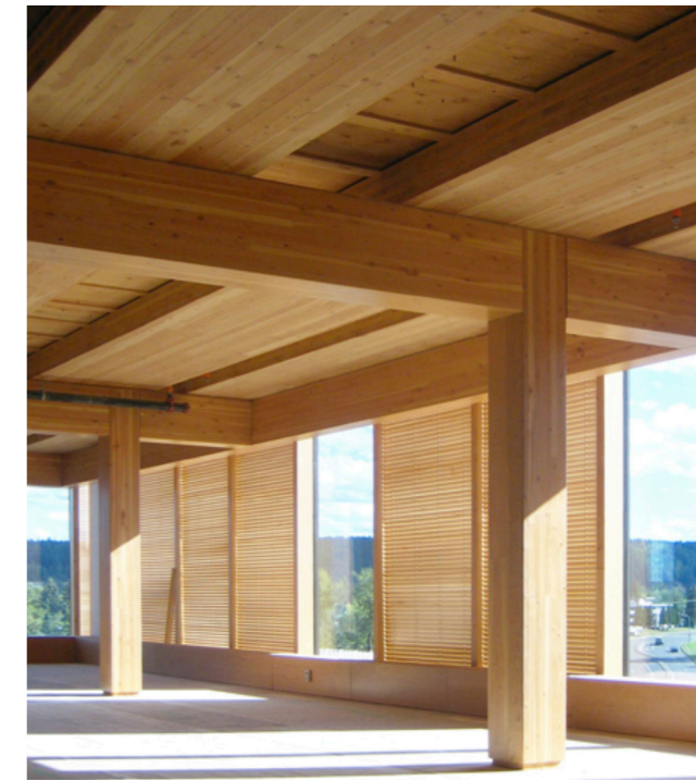
Main Structure: CLT Wood
