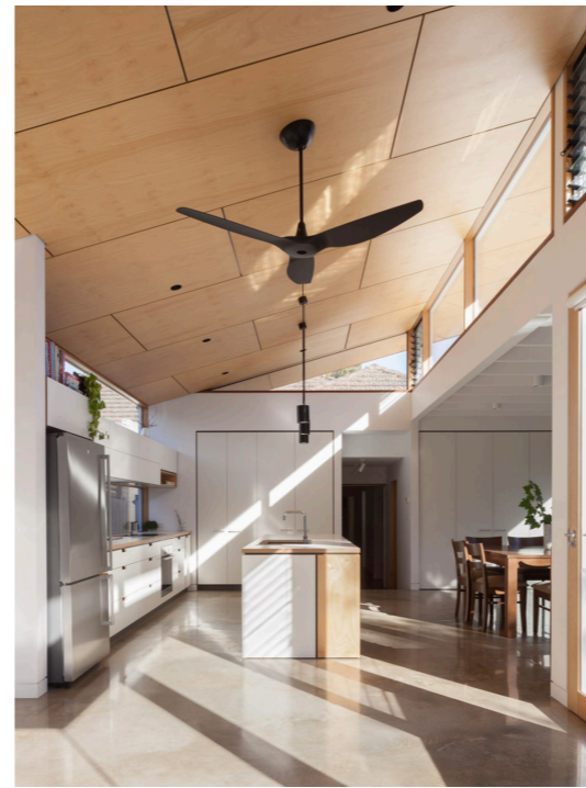
Exterior and Interior Ceiling: Fir-Faced Plywood
