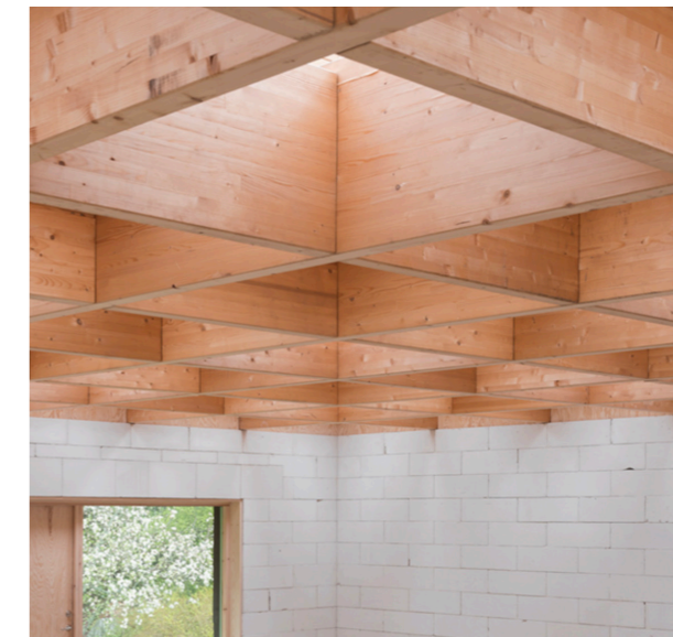
Landscape Roof Structure: CLT Waffle
