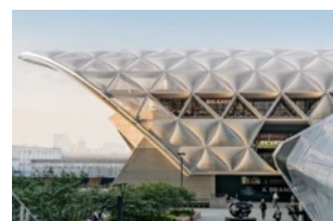
Figure 40 – Canary Wharf Crossrail Station, London. Facade from light, air-filled ETFE foil. Designed by Foster + Partners planned to be finished in 2021
