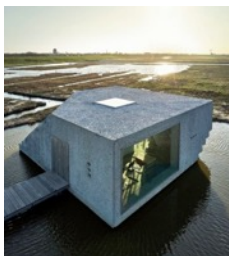
Figure 35 – Office Natuurmonumenten Zierikzee made of the thermal insulating warmbeton. Designed by Architectenbureau Rink Tilanus
