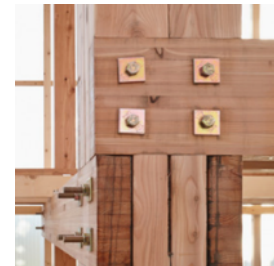
Figure 62 – Accessible and detachable wooden connection (Durmisevic et al., 2019)
