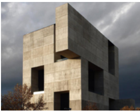
Figure 41 – Innovation centre University of Santiago. 14-storey building made of reinforced concrete with monolithic concrete finish
