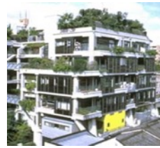
Figure 30 – Next21, an experimental housing development using open building principles in Osaka, Japan. Designed by SHU-KO-SHA in 1994
