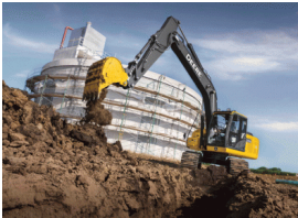
Figure 36 – Excavator during earthmoving on construction site
