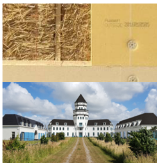
Figure 42 – Country house Zoutelande. This traditionally looking building, is not traditional. It is self-sufficient and made of bio-based materials such as wood, straw, loam, and lime. Designed by ORIO architecten
