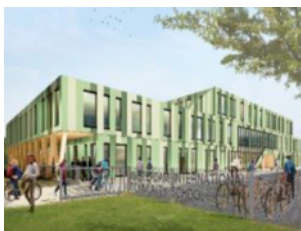
Figure 32 – AIC School. This 100% modular building supposed to be finished in 2020 and be disassembled and reused 5 years later. Designed by BurtonHamfelt Urban Architecture
