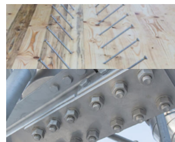
Figure 45 – Bolted steel in load bearing structure (top) & dry joints in wooden load bearing structure in (down, Triodos III, Zeist)
