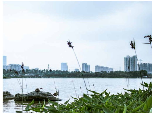
FIG. 4.6 New town construction based on Haizhu Lake / Source: Author
