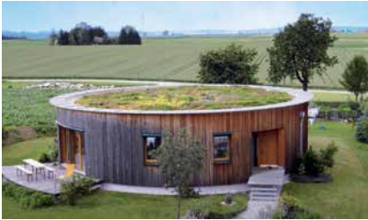
FIG. 3.2 A round passive house floorplan resulting in a favourable shape factor
