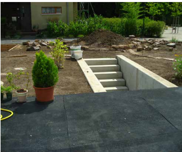
FIG. 3.5 A separate entrance into the unheated basement underneath the building (view from the terrace during construction)
