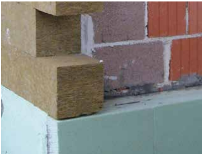
FIG. 4.1 A+B+C: A massive wall – brick with external mineral wool and XPS thermal insulation
