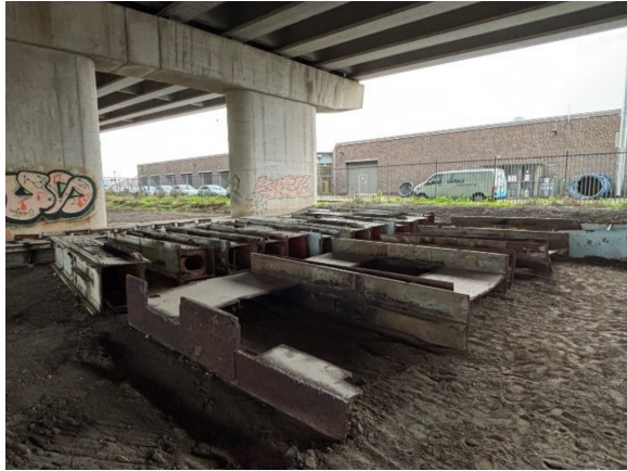
(a) Dismantled steel members from the Old Botlek Bridge at the storage site.
