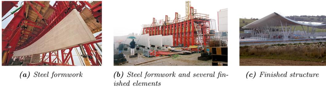
**Figure B.3:** Millau viaduct toll gate (Structurae, 2005)
