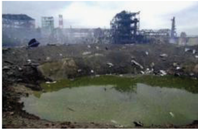
Fig 6 – the crater left by the explosion of ammonium-nitrate at the AZF fabric of Toulouse (from B. Cahen 2006)
