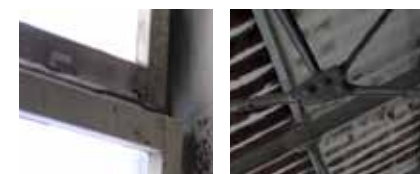
Wooden window frames Steel roof construction
