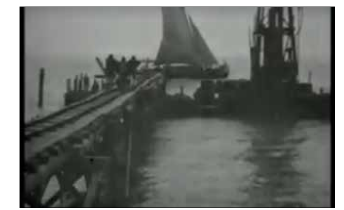
(2) Pier with rails (B)
