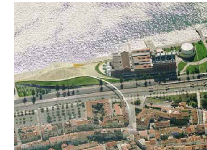
(2) Museum of Electricity 2006 - Area of Belem
