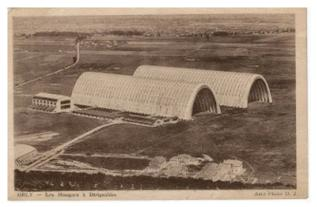
The airship hangers at Orly, France were built by Eugene Freyssinet between 1921-1923. The program which Freyssinet needed to follow stipulated that a sphere with a radius of 25 meters had to fit, unobstructed, within the hangar. The buildings dimensions were carefully determined so that they could house the airships without much extra space resulting in unneccesary additional costs and building stresses. The hangars were destroyed in WWII by American aircraft.
