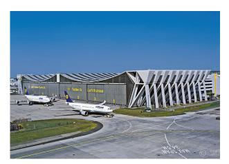
The Lufthansa Maintenance Hangar V at Frankfurt Airport has a spectacular form that results directly from the load-bearing structure, which consists of two suspended roofs. The thin prestressed concrete bands forming the roof surface are supported by cables spanning between large truss-like support structures..
