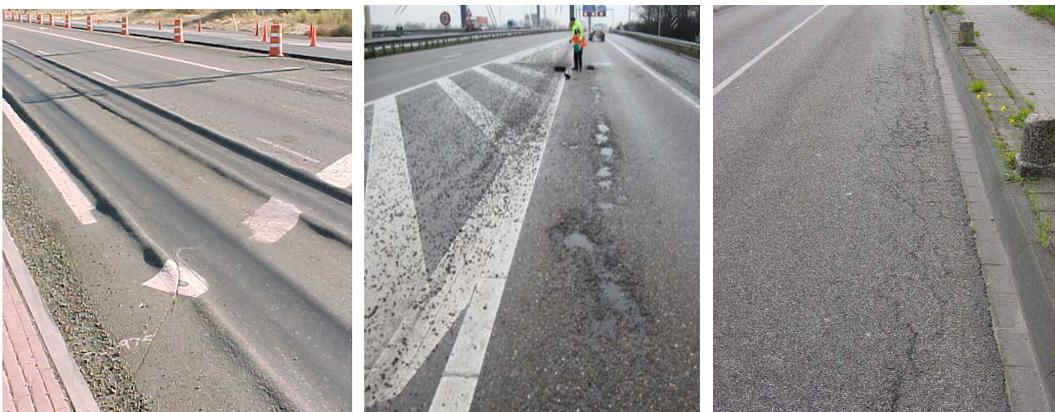
Figure 1-1 Rutting, disintegration and cracking in pavements [13, 16, 17]
