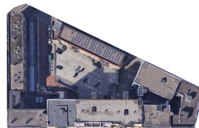
big openings - parking lot
