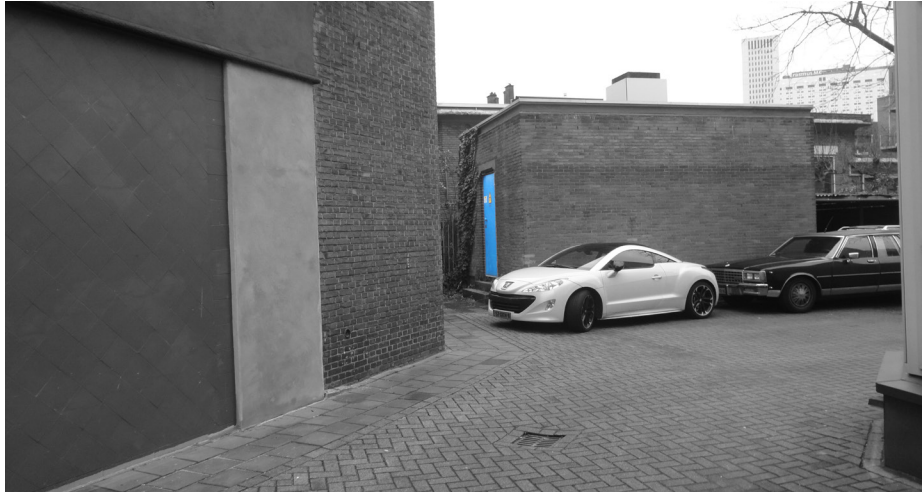
03.a.d. The striking blue door warning for electricity danger
