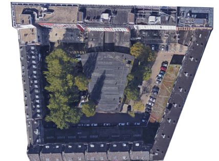
ground floor openings- parking lot
