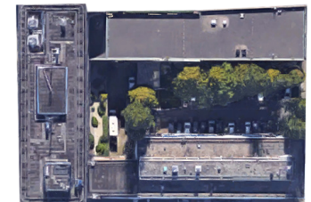
one side open-parking lot
