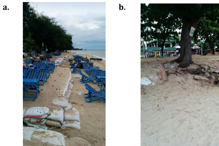
Figure 2.1 | Problems at Cha-am. (a) Narrow beach at Cha-am, locals have placed sandbags along the beach in an effort to stop the erosion. (b) Steep beach at Cha-am with sandbags emplaces by locals visible, the situation around the tree shows that the beach is receding. Some waste is also visible, which is a problem at Cha-am beach (own pictures).
