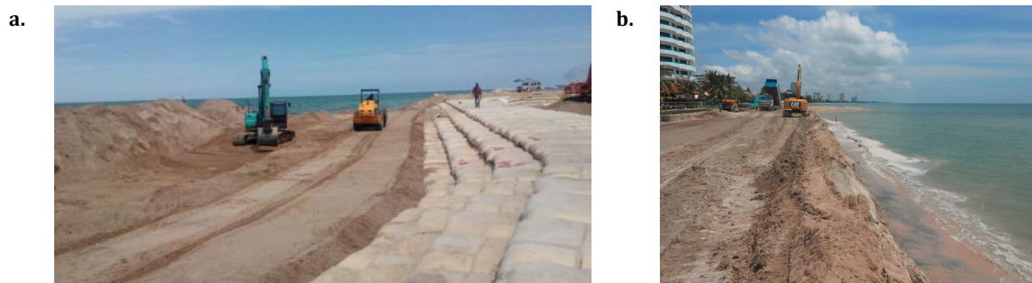
Figure 7.2 | Constuction of geotextile revetments (source Marine Department, 2016)
